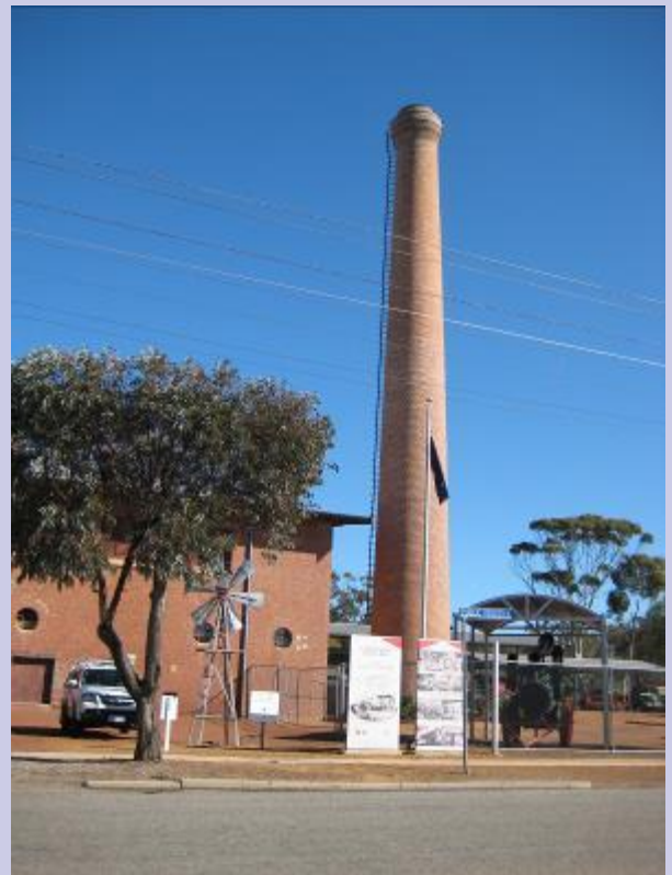
Cunderdin Museum Pump Station No. 3
