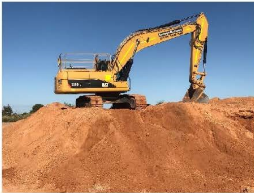
DRIVEWAYS, CARPARKS & YARD WORKS
