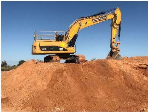
DRIVEWAYS, CARPARKS & YARD WORKS
