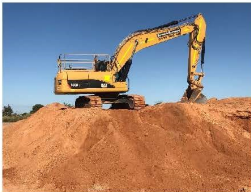
DRIVEWAYS, CARPARKS & YARD WORKS
