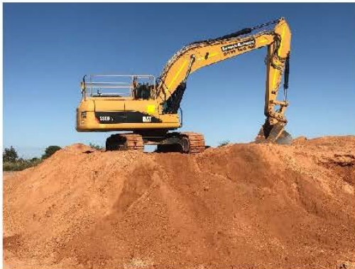
DRIVEWAYS, CARPARKS & YARD WORKS
