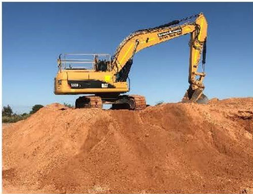
DRIVEWAYS, CARPARKS & YARD WORKS
