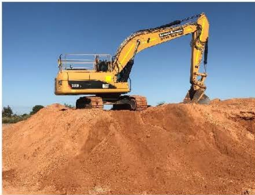
DRIVEWAYS, CARPARKS & YARD WORKS
